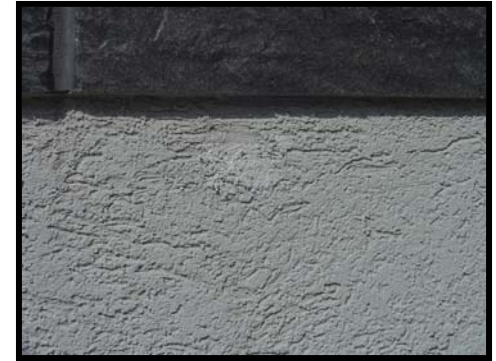
Stucco may appear the wrong color at first but once it dries it will look identical.
