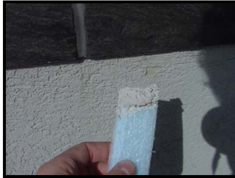
Using a paint brush, foam piece or finger swirl in the stucco.
